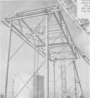
THE FOURTEEN-ton truss section of Lago's new pipe bridge was erected by the contractor March 19 with the aid of Lago's two heavy-duty cranes. Forty-foot columns support the section. E SECTION di aguanté di dies-cuatro ton na e brug nobo di tubo na Lago a wordé crui door di e contratista Maart 19 cu ayudo di dos grusaan piá di Lago. Columnanan di cuarenta pia ta wanta e seccion.
